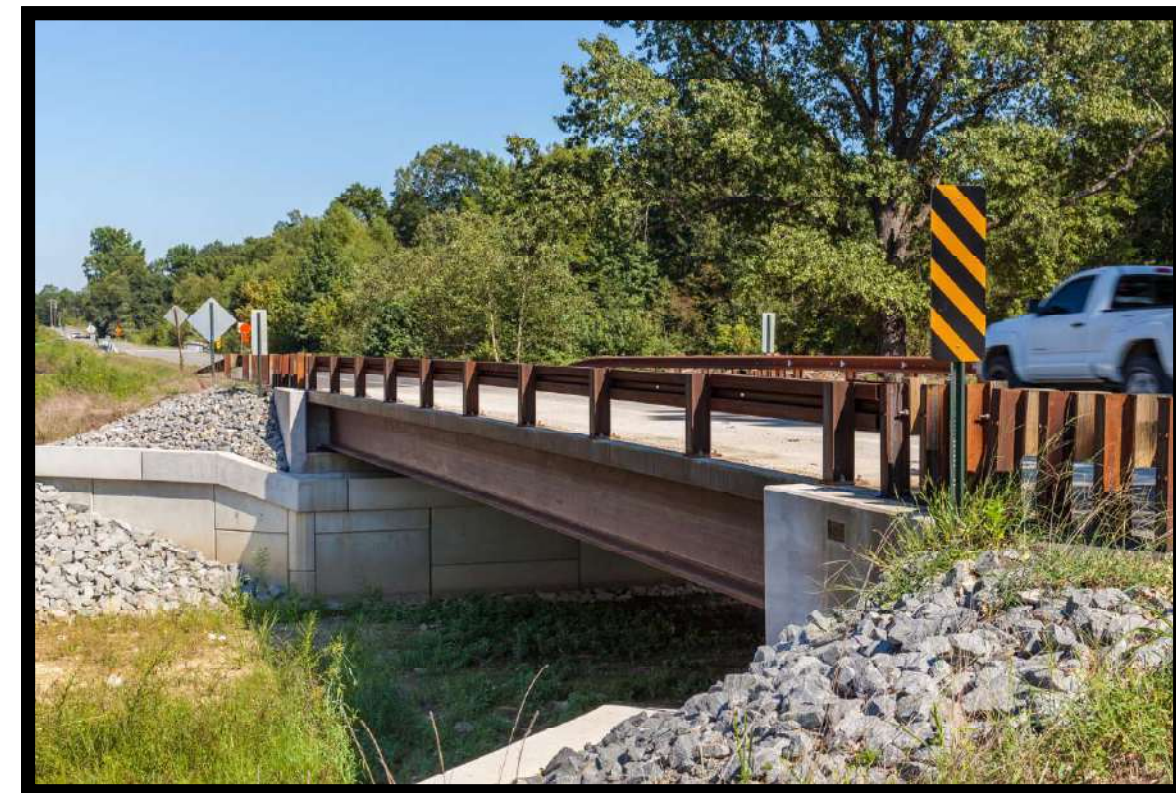
Algonquin Vehicular Girder Bridge
