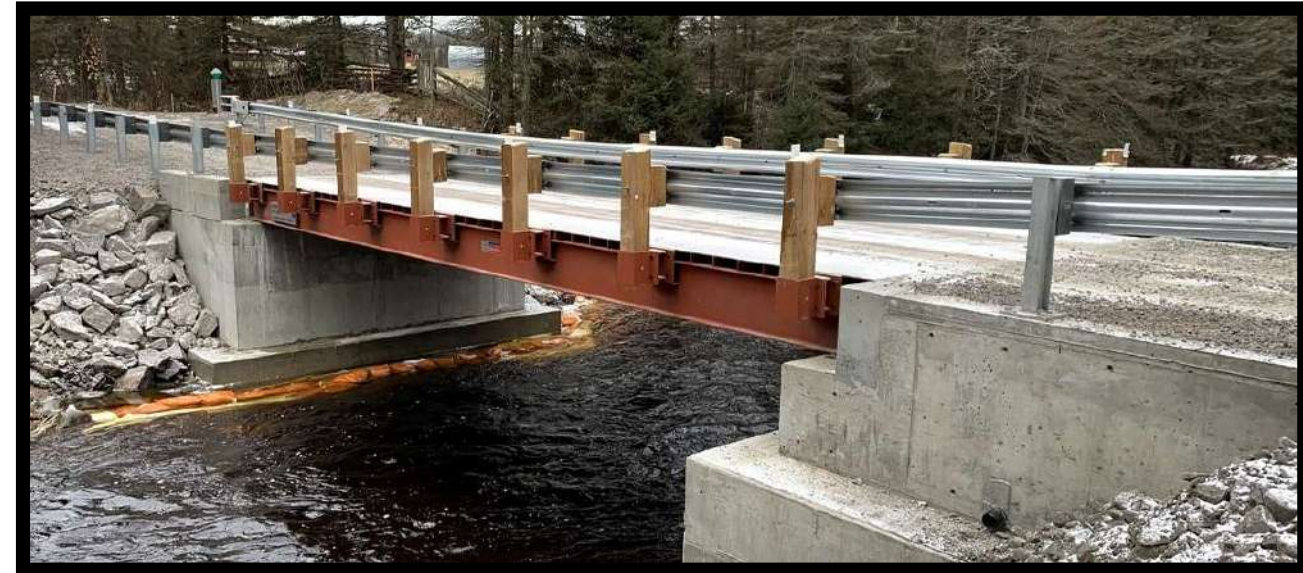
Northern Mat & Bridge Municipal Modular Access Bridge
